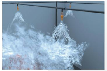
**External sprinklers** – a system of sprinkler heads provided along an external wall to protect the building from external exposures such as another building or yard storage.
