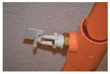
**Fast response sprinkler** – has a high level of thermal sensitivity which enables it to respond at an early stage of fire development.
