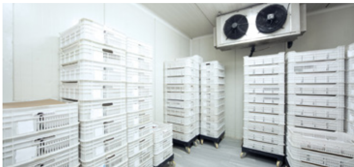
Cool room - EPS construction
