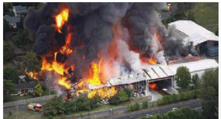
Fire involving EPS panels
