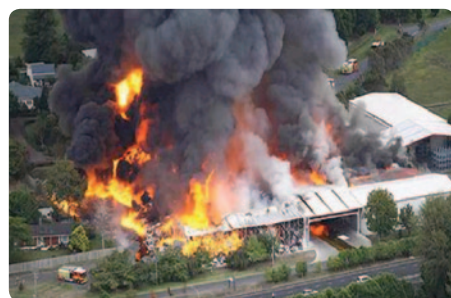
Fire involving EPS panels
