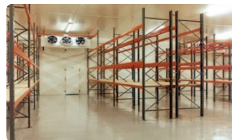
Cold room storage – insulated with EPS panels, walls and ceilings
