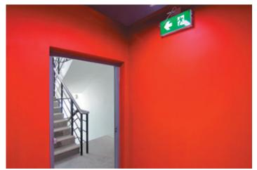
Due to the number of components needed to effectively address a penetration or barrier, each of the following is termed a system. For example, a fire resistant doorset requires a fire-resistant door leaf, frame and furniture, commonly referred to as hardware. These items make up a doorset and therefore the system.
